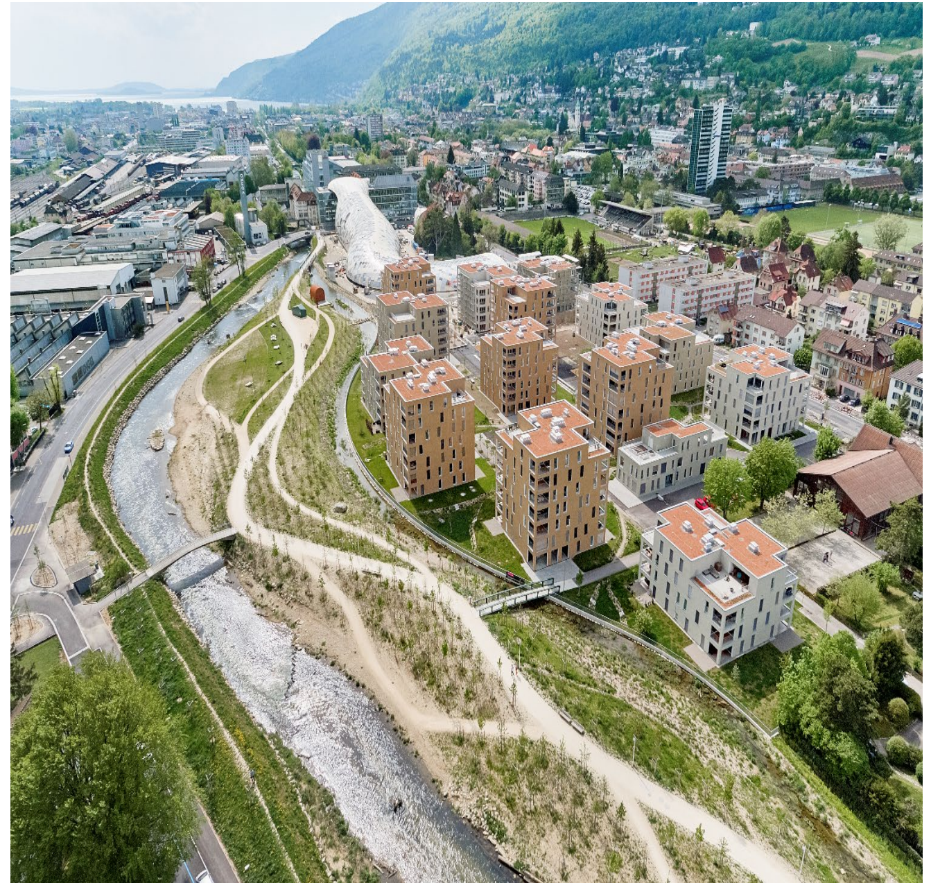
Project completion: 2018 - Client –Previs Pension Fund - Jardin du Paradis
